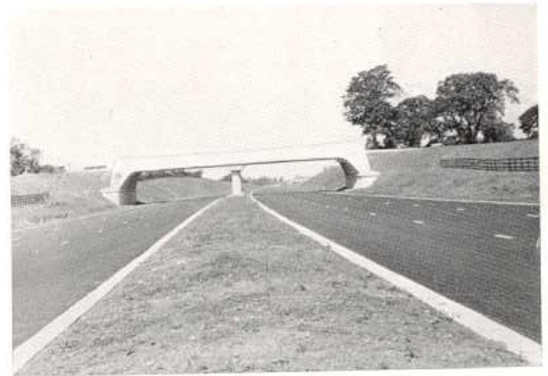
The London - Yorkshire Motorway at Rothersthorpe
